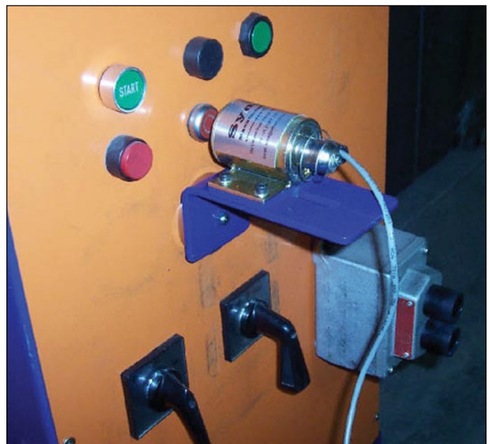
Figure 1 — Remote breaker trip actuator with magnetic base
