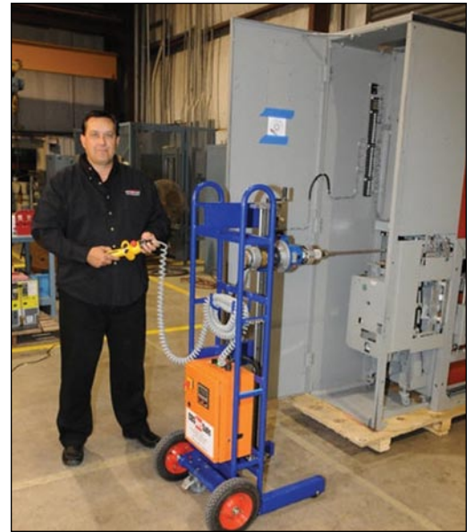
Figure 2 — Trying out a remote breaker racking device at our shop
